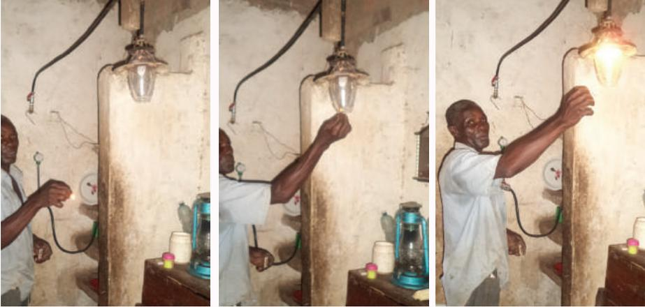
*Fig. 9 lighting the biogas*
