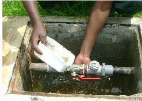
**Fig. 5 Testing for gas leakage**
