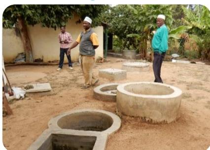
**Ramadan Sungu** is a local Islamic leader and an influential person. He was also the first in his village to adopt the biogas technology, and in order to have a maximum gas and slurry production, he even connected one of the toilets. He uses the bioslurry for his fishponds, fodder production and for the cultivation of carrots, beans, peas, cassava, rice, maize, ground nuts, sunflowers
